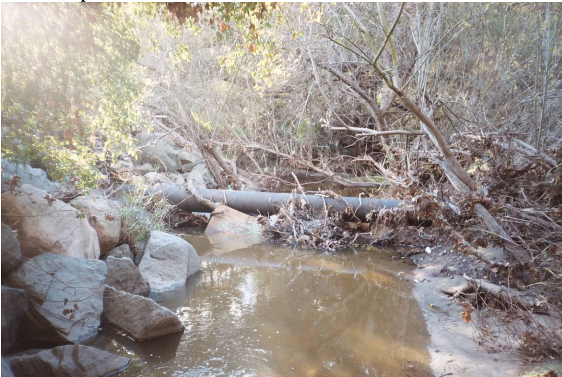
SR2-4b – exposed sewer line in 2005
