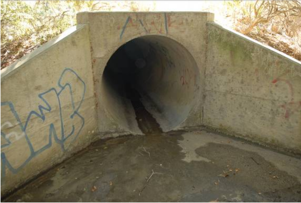
SR2-3a – culvert outfall in 2008
