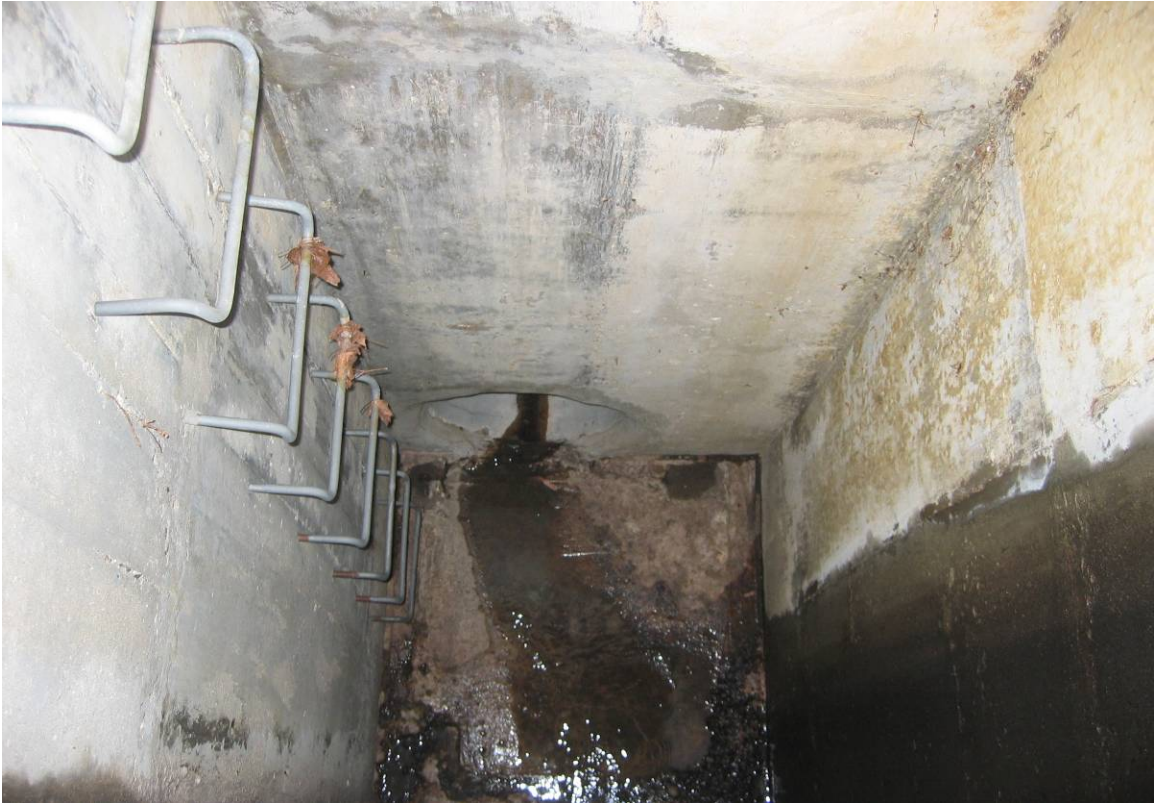
SW2-1 – storm drain
