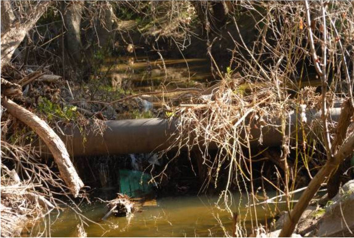
SR2-4b – exposed sewer line in 2005
