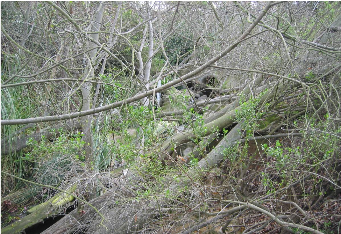
SW2-2 – storm drain outlet
