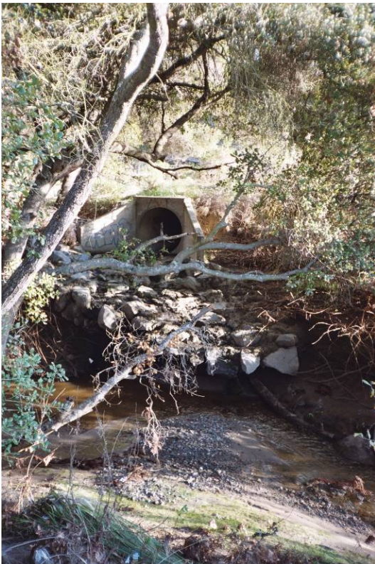
SR2-3b – culvert outfall in 2004
